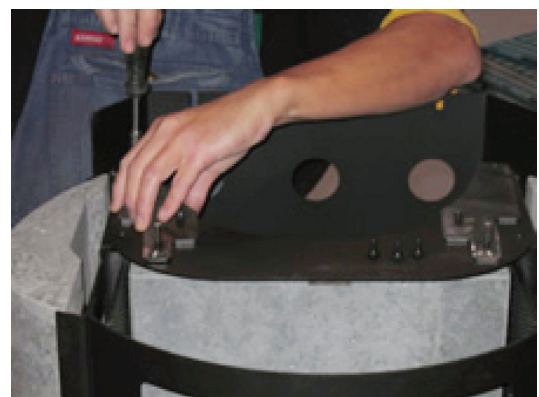
25. Attach the two brackets supplied.
