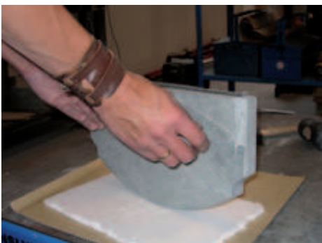
21. Protect the stones during installation.
