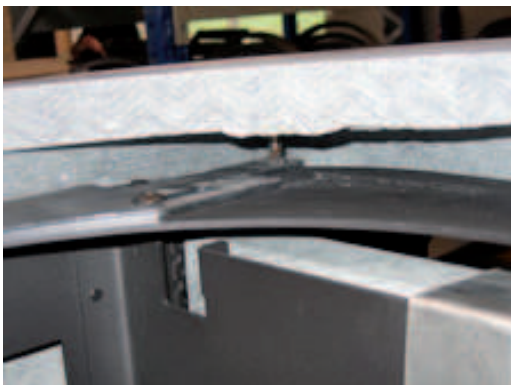
29. Rear view of the installed top panel.
