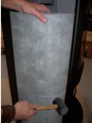
11. Use a rubber mallet to gently adjust the sides so there are no gaps.
