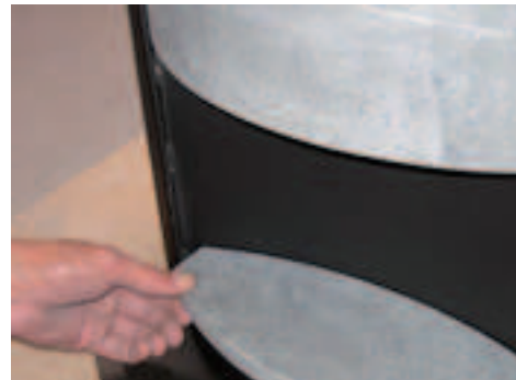
39. Place the base stone at an angle inside the ash door and rotate into position.
