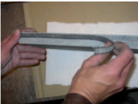
20. Before installing the horizontal stone, attach the sealing strip provided to the back.
