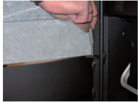
38. Once the stone is in place, carefully re-tighten the screws so that the stone cannot move.
